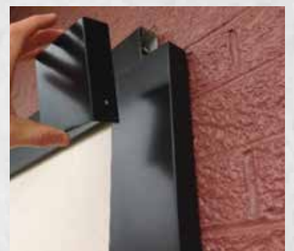
Install corner and seam covers
