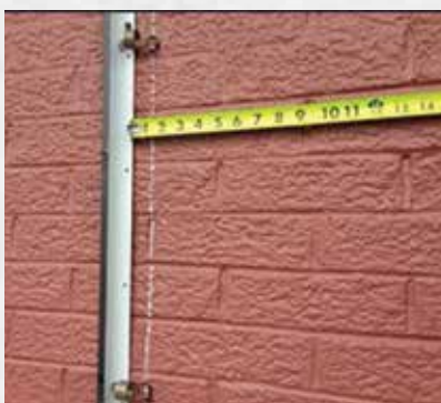
Install sign frame bracket
